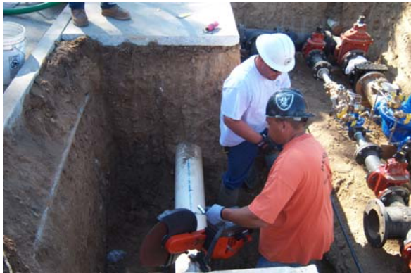
Cutting of KID 8" PVC Main for Interconnection
