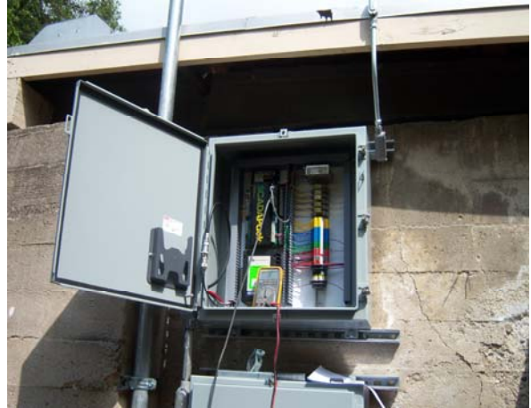
Brown Reservoir SCADA Installation
