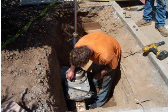
Line Stop to Facilitate Interconnection
