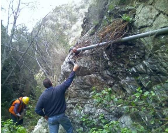
Delores Tunnel Pipeline Repair
