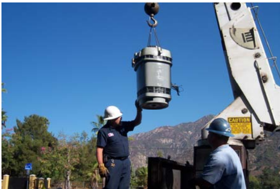
K-3 Well Motor Repair
