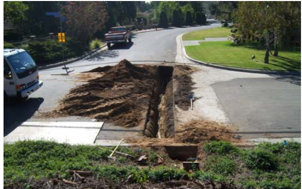
Replace Villa Knolls Service Lines
