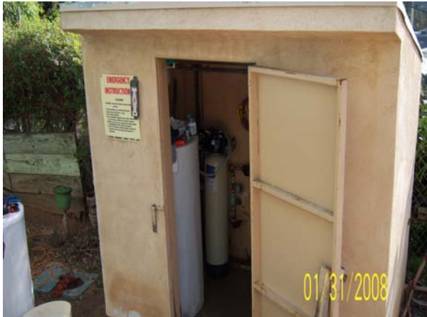
Holly Chlorinator Building
