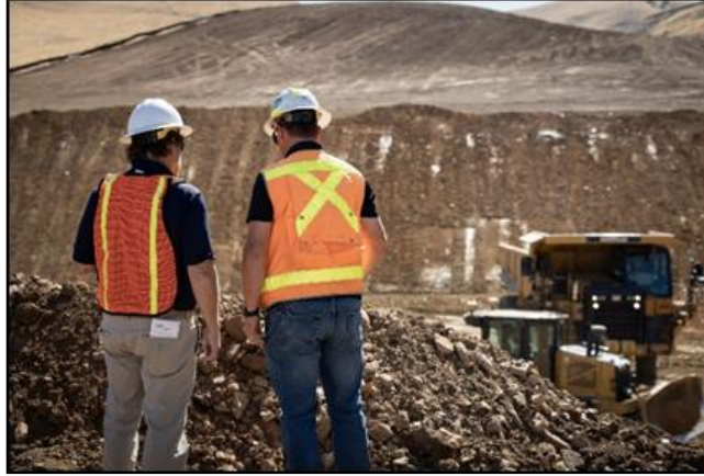
Figure 2. IIJA-Funded Bureau of Reclamation B. F. Sisk Dam Safety Construction Project
