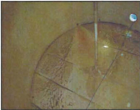
Interior - Before Washout
