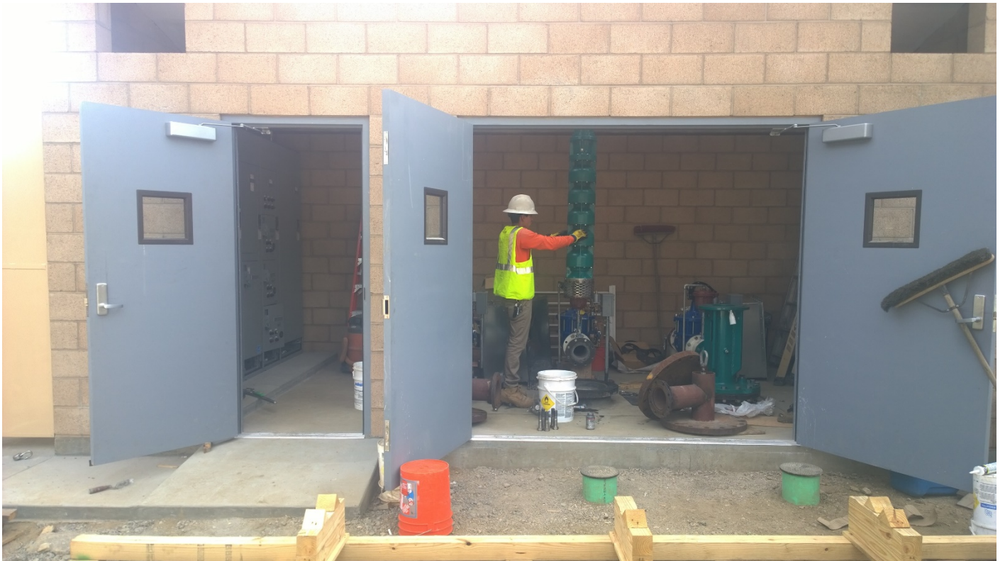
Installing Booster Pump #2
