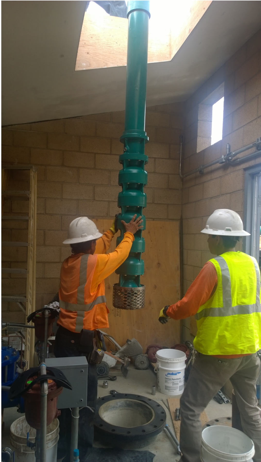
Lowering Booster Pump #1 through Skylight
