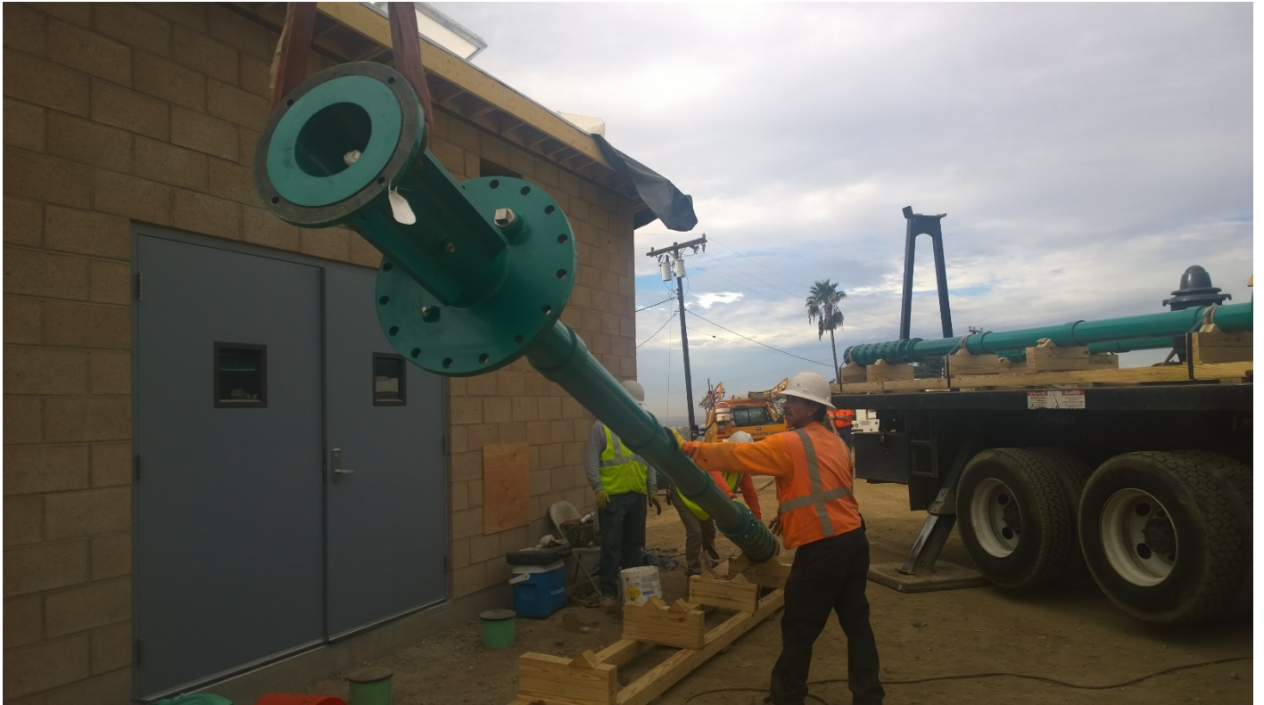
Unloading Booster Pump #1
