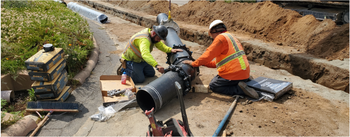
Kinneloa crews install a new water main.
