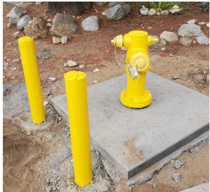
Newly installed fire hydrants enhance public safety.
