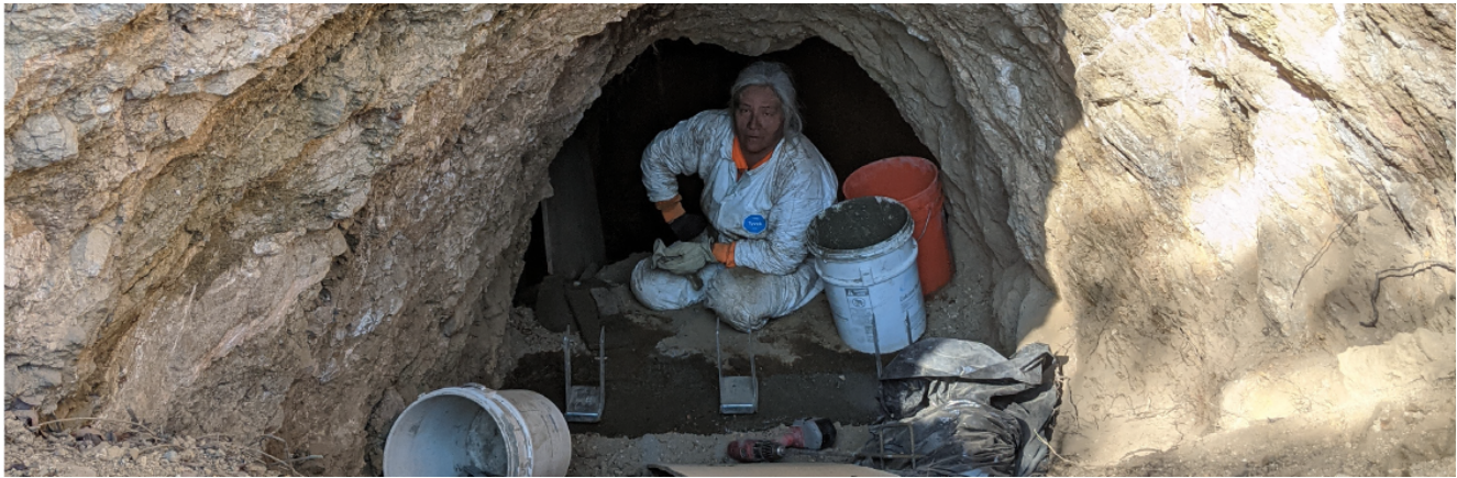
Crews work inside the House Tunnel to restore water service.
