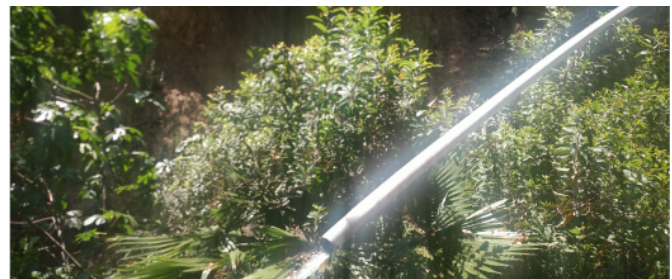
The restored House Tunnel provides a steady stream of water.
